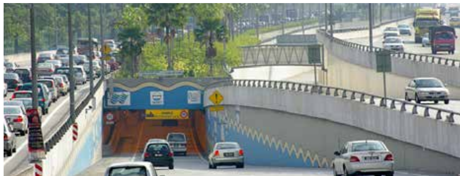
Malaysia's SMART Tunnel (Stormwater Management and Road Tunnel) is an example of resilient infrastructure that handles traffic congestion and also diverts water in storm events
