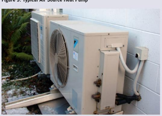
Figure 9: Typical Air Source Heat Pump
