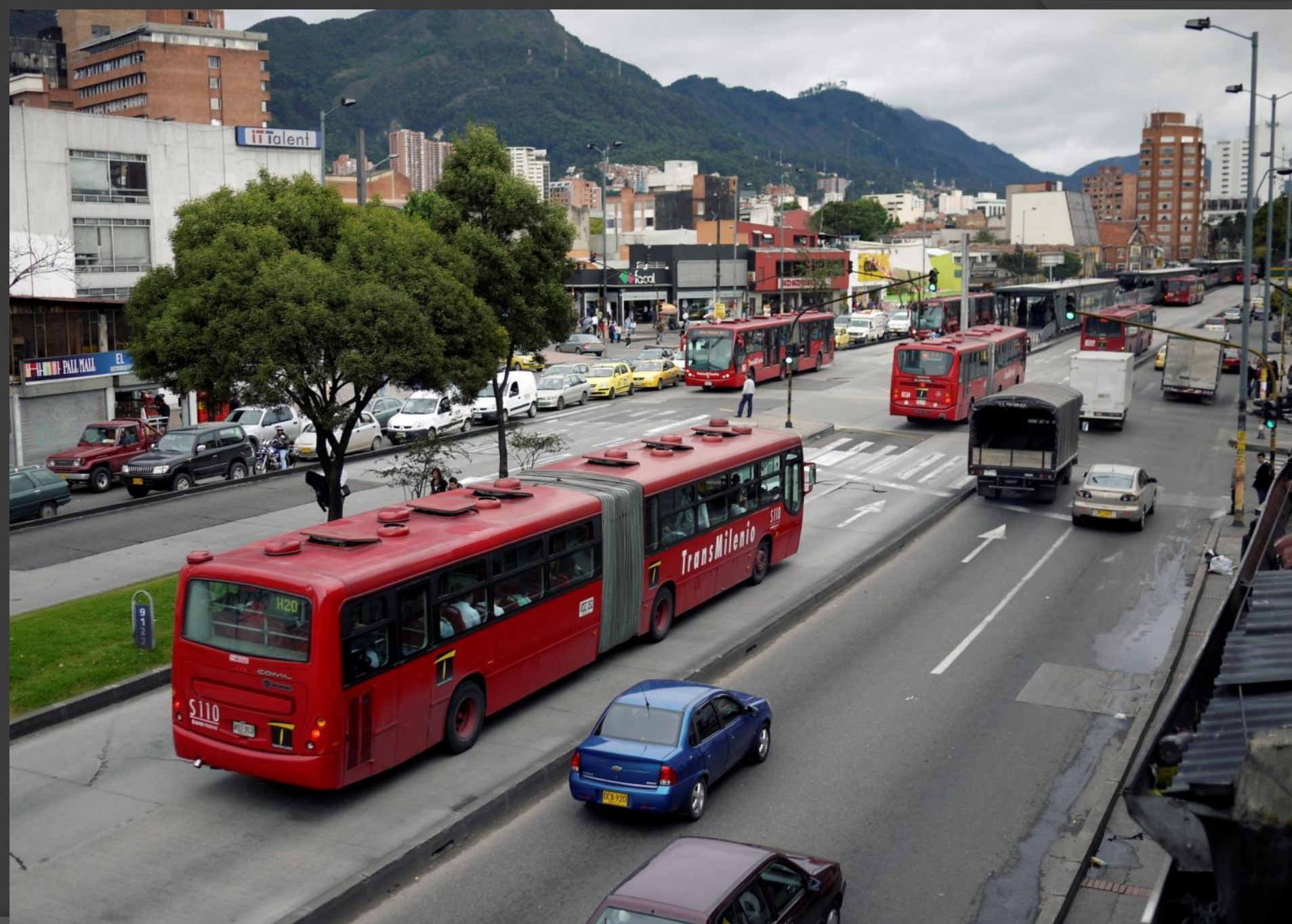
BRT in Bogota – highest throughput point in the system: only 36m wall-to-wall
