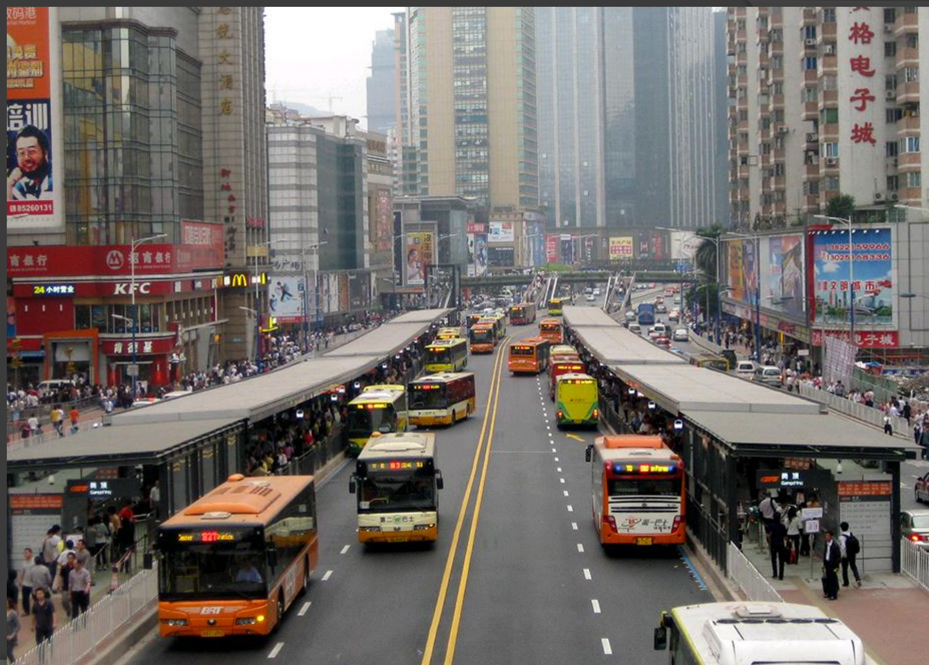
Gangding BRT station, after the BRT implementation
