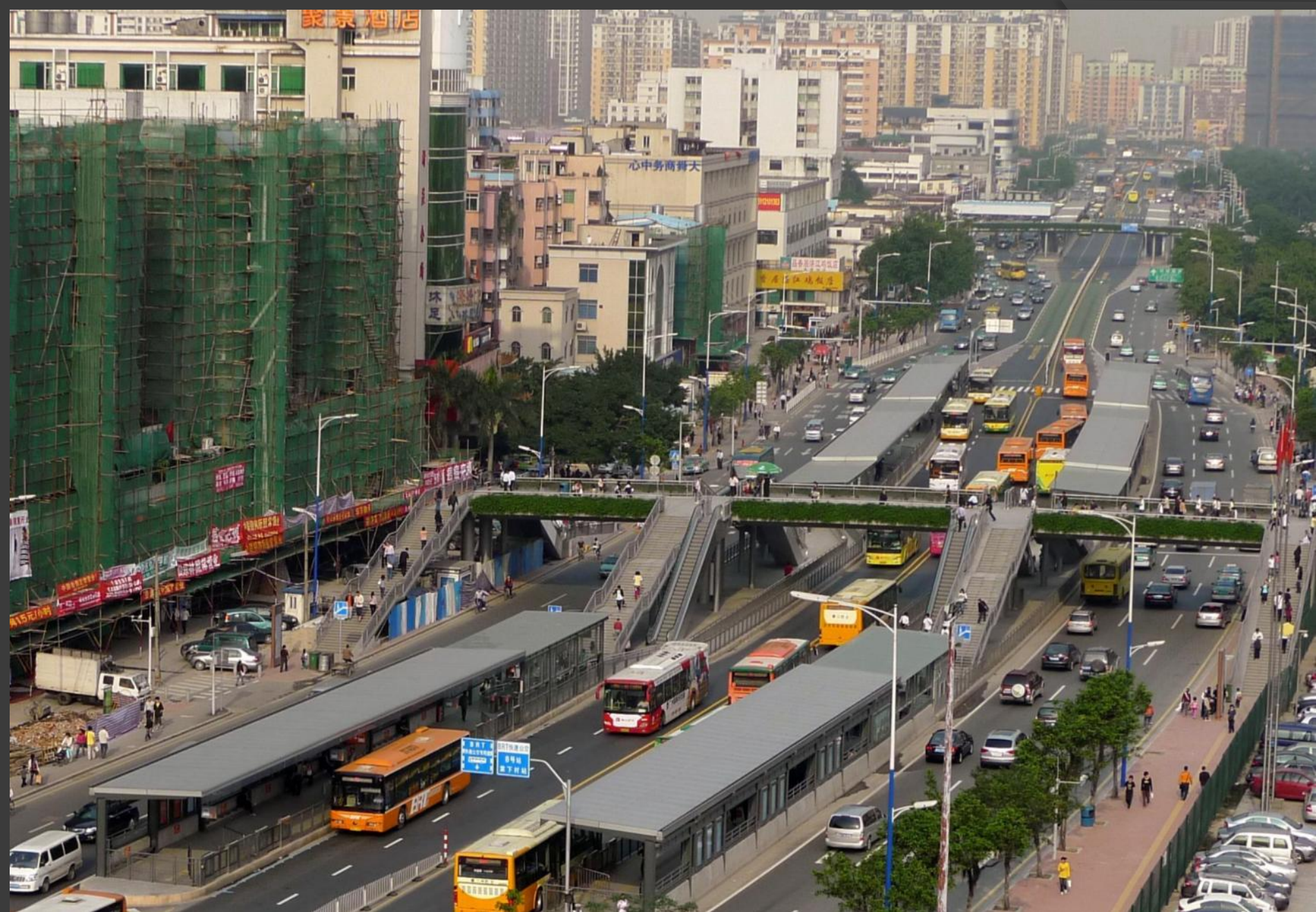
3 substops, Tangxia station. Tangxia station has around 8,500 passenger boardings in a single hour during the morning peak. Station access is via a bridge with escalators, and a pedestrian crossing with refuge islands
